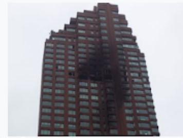
The Belaire building after the fire caused by the crash was extinguished
