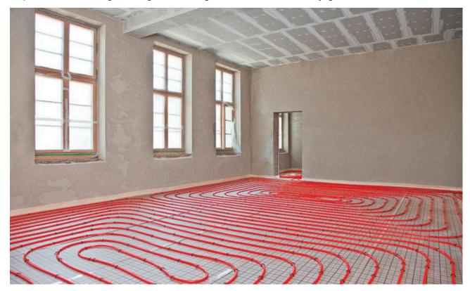
Another advanced alternative to conventional HVAC systems is the slab cooling and heating system. This method involves embedding water pipes into concrete slabs, allowing the building's thermal mass to regulate indoor temperatures. By using the natural cooling and heating properties of concrete, slab cooling and heating system provide consistent, energy-efficient temperature control throughout the day.
