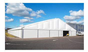
Warehouse tents are structures that are erected quickly and are designed to protect your goods from the elements. They are constructed from metal frames and waterproof fabric, making them an ideal solution for outdoor storage. The metal frames are designed to
