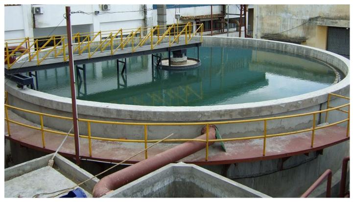
are suitable for tanks up to 50 meters in diameter. The clarifier has a special drive unit that is fitted to the shaft or cage. This cage or shaft can be provided with an overload sensor if required by the client. By means of the shaft or cage, scraper arms with scraper blades are connected to the drive unit.
