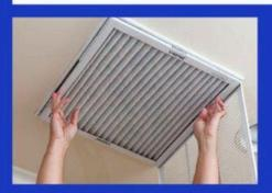
Replace or clean the furnace filter every 1-3 months to ensure efficient airflow and maintain indoor air quality.
