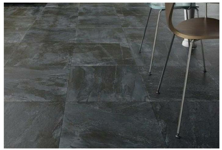
Slate is much more fire resistant and able to sustain temperatures higher than many metals. It works well for surfaces like floors and roofs because it can withstand extreme temperature changes.
