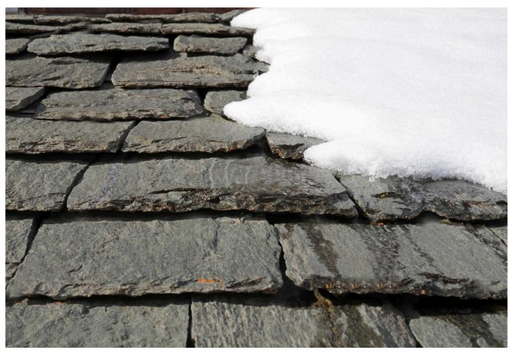
Slate is especially well suited for roofing because it has a very low water absorption index—less than 0.4 percent—which makes it resistant to damage from frost. The embodied energy of natural slate, which needs no processing, is comparable favourably to that of other roofing materials.
