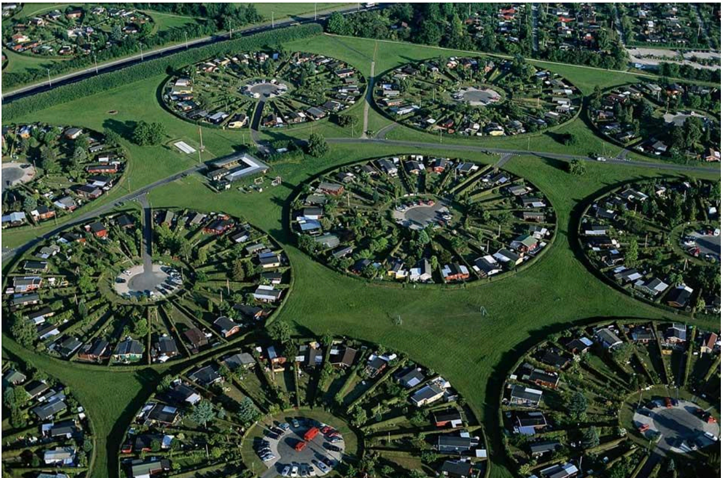
Suburbs of Copenhagen, Denmark
